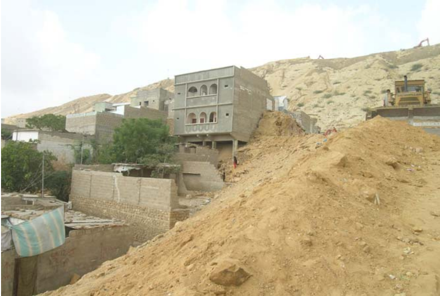
North Nazimabad and Qasba Colony Link Road: The community was awarded compensation at market value for their houses. (February 28 th 2007 View from North
