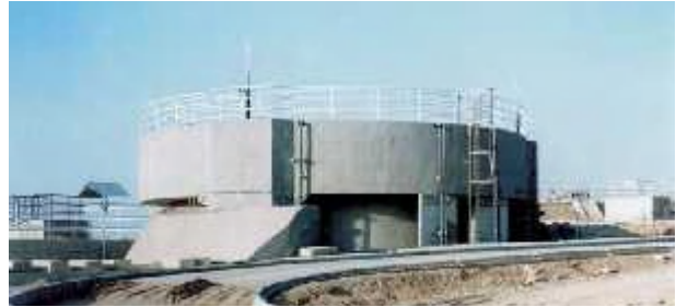
HUB WATERTREATMENT PLANT - C4
