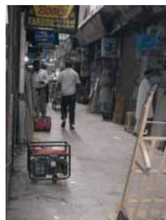
Lined up generators outside the shops in Urdu Bazaar
