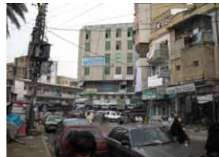
Jumbled up overhead wires and Kunda's can be seen all the market
